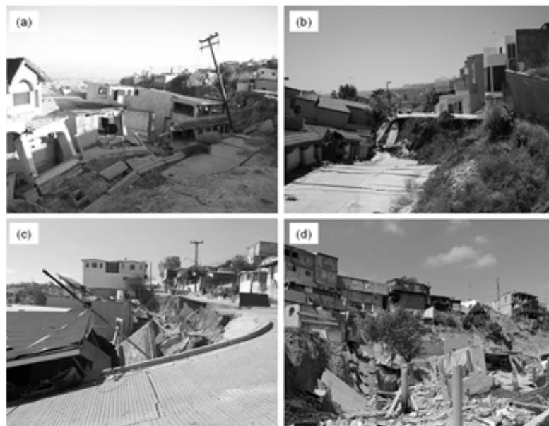
Figure 1. Some urban landslides occurred in Tijuana.
