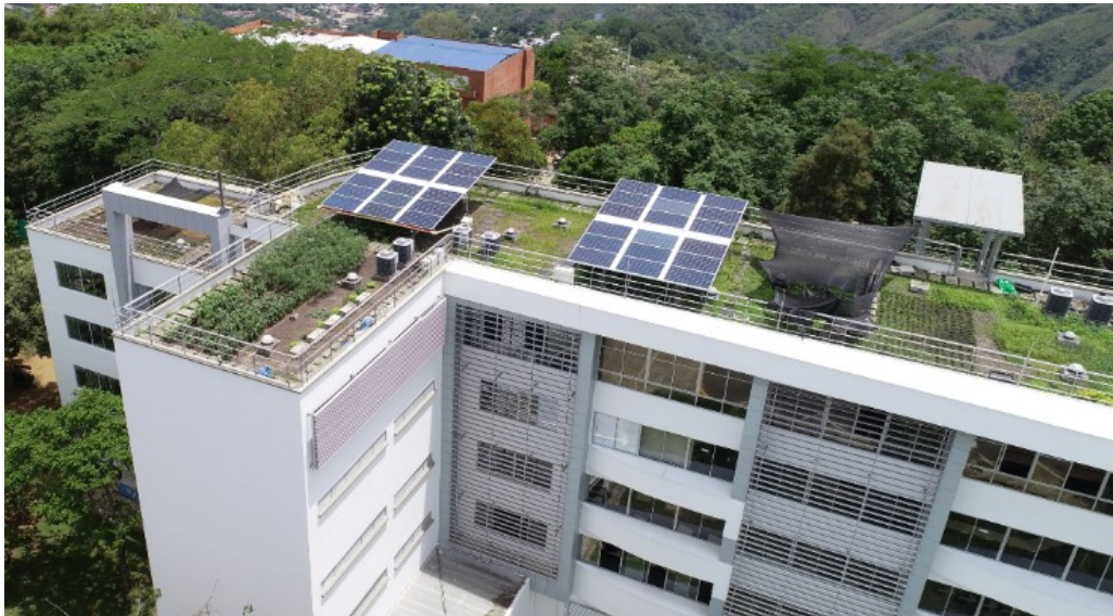
Figure 3. Electrical Engineering Building
