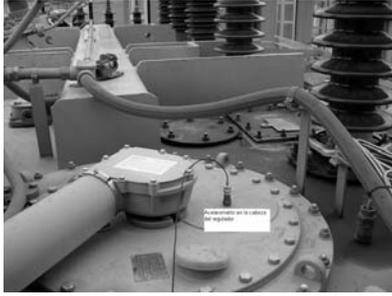
Figure 4 Accelerometer located on the OLTC head
