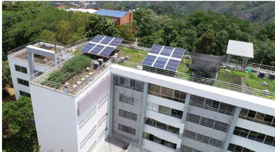
Figure 3. Electrical Engineering Building
