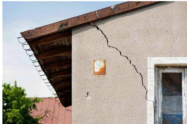
Figure 2. Earthquake-induced cracks (WebAdictos, 2017).
