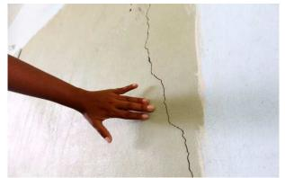
Figure 6. Cracks in the wall (Ayala, 2017).
