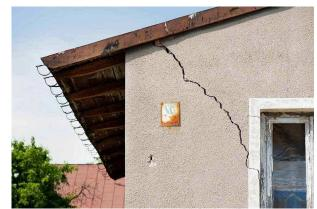
Figure 2. Earthquake-induced cracks (WebAdictos, 2017).
