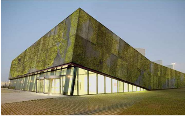
Figure 1. Multilayer concrete developed by the Universitat Politècnica de Catalunya (Staff, 2017).
