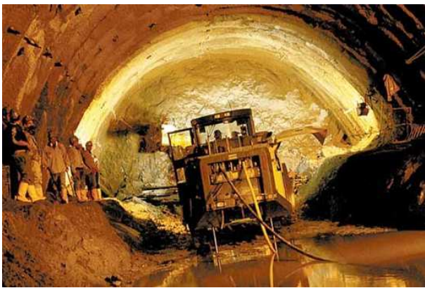
Figure 4. Works in the La Linea tunnel (El Espectador, 2017).
