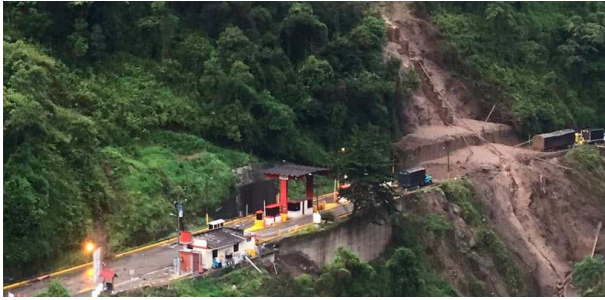
Figure 10. Work to enable the passage through La Línea (Invias, 2017).
