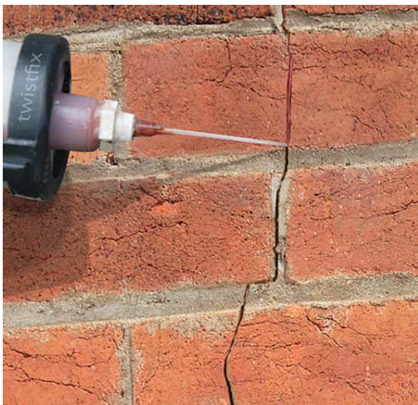
Figure 4. Brick repairs (Brick Repairs, 2017).
