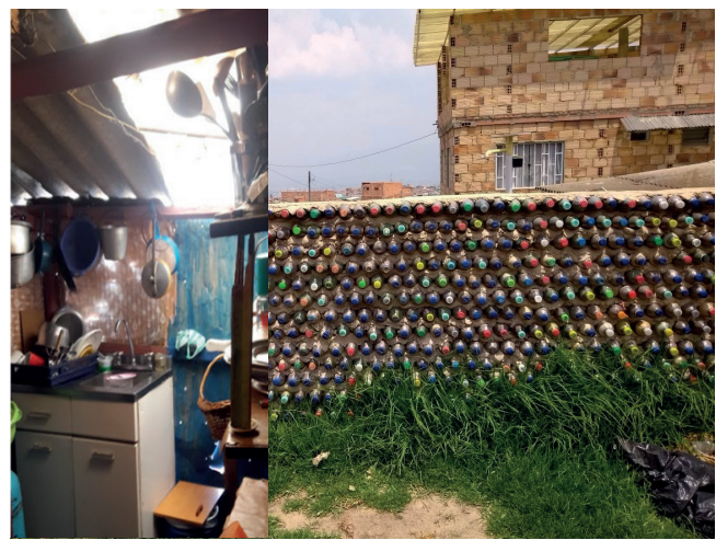
Figure 5. Light litre and Community room wall [18].
