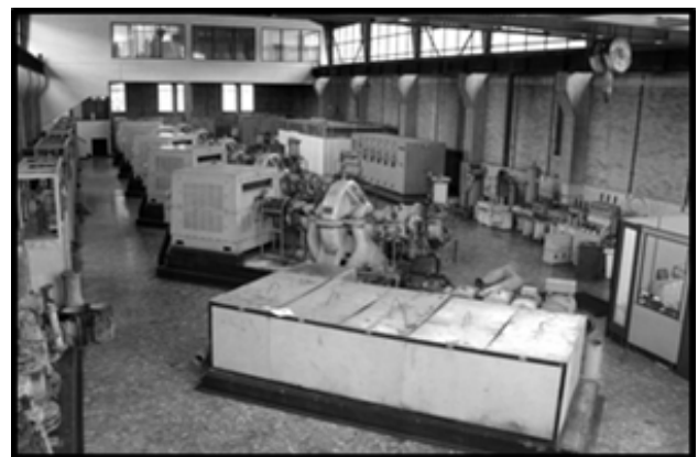
Figure 3. Usaquén Pumping Station [21].
