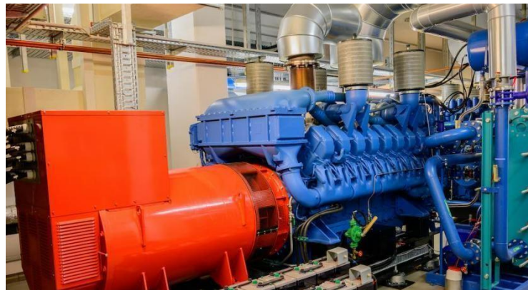
Figure 1. Diesel Generator. [4]
