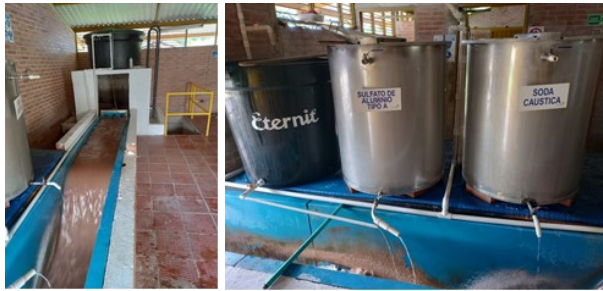
Figure 2. a) Rapid mixing (Parshall flume) b) Tanks with Coagulant and pH Corrector.
